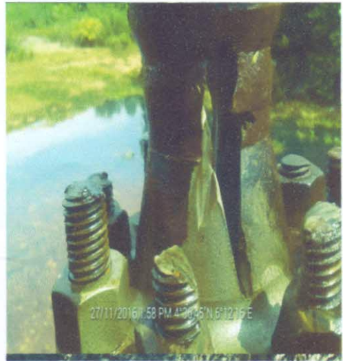
SPILL POINT AFTER REPAIRS: fig4
